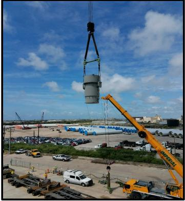
Once the Reactor Pressure Vessel was secure in its specially designed shipping container, it was lifted out of the STURGIS and loaded onto a transport vehicle for shipment to Waste Control Specialists, the selected disposal facility.
