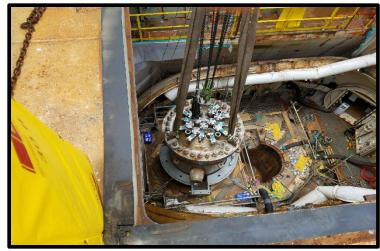
Reactor Pressure Vessel is lifted and placed into a specially designed shipping container to its left within the Reactor Containment Vessel.
